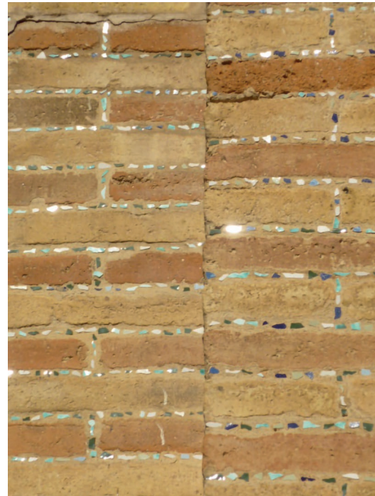
▪ Fig. 9. Antoni Gaudí. Part of the wall with bricks and trencadís in the joints. 1884-87. Photograph of the author.
