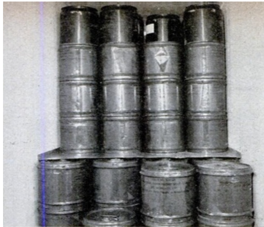
View of inside of bin shows stacked cans of Glauber's salt that actually store the heat. Closetlike bins are closed off from rest of house and need to be opened only for adjustments.
