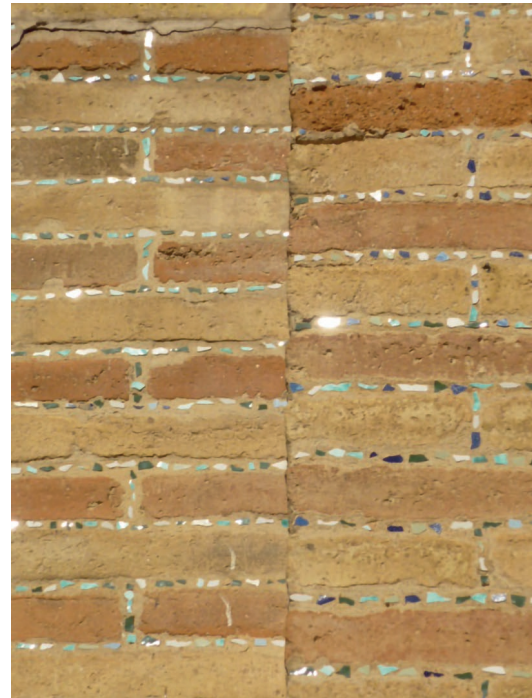
▪ Fig. 9. Antoni Gaudí. Part of the wall with bricks and trencadís in the joints. 1884-87. Photograph of the author.
